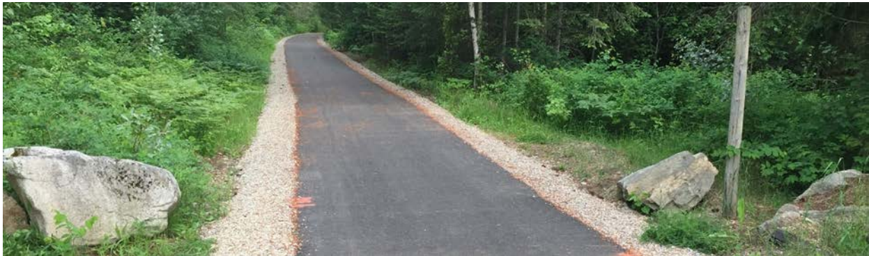
Type 1 Trail, Hard Surface tread sample – South Slokan Rail Trail
