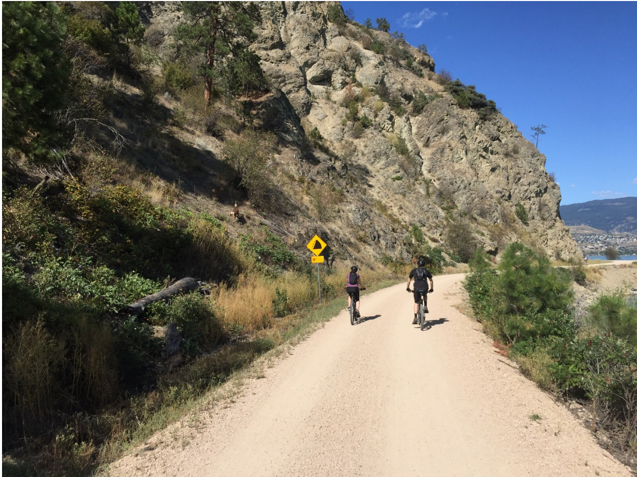
Type 2 Trail, highly compacted aggregate surface tread – Okanagan Rail Trail
