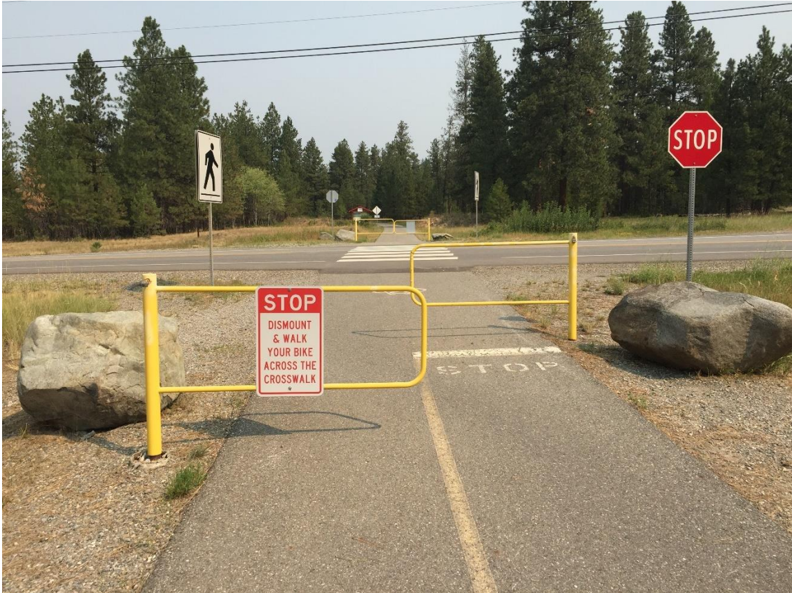
Example of baffle gates. (North Star Rail Trail, Kimberly to Cranbrook)
