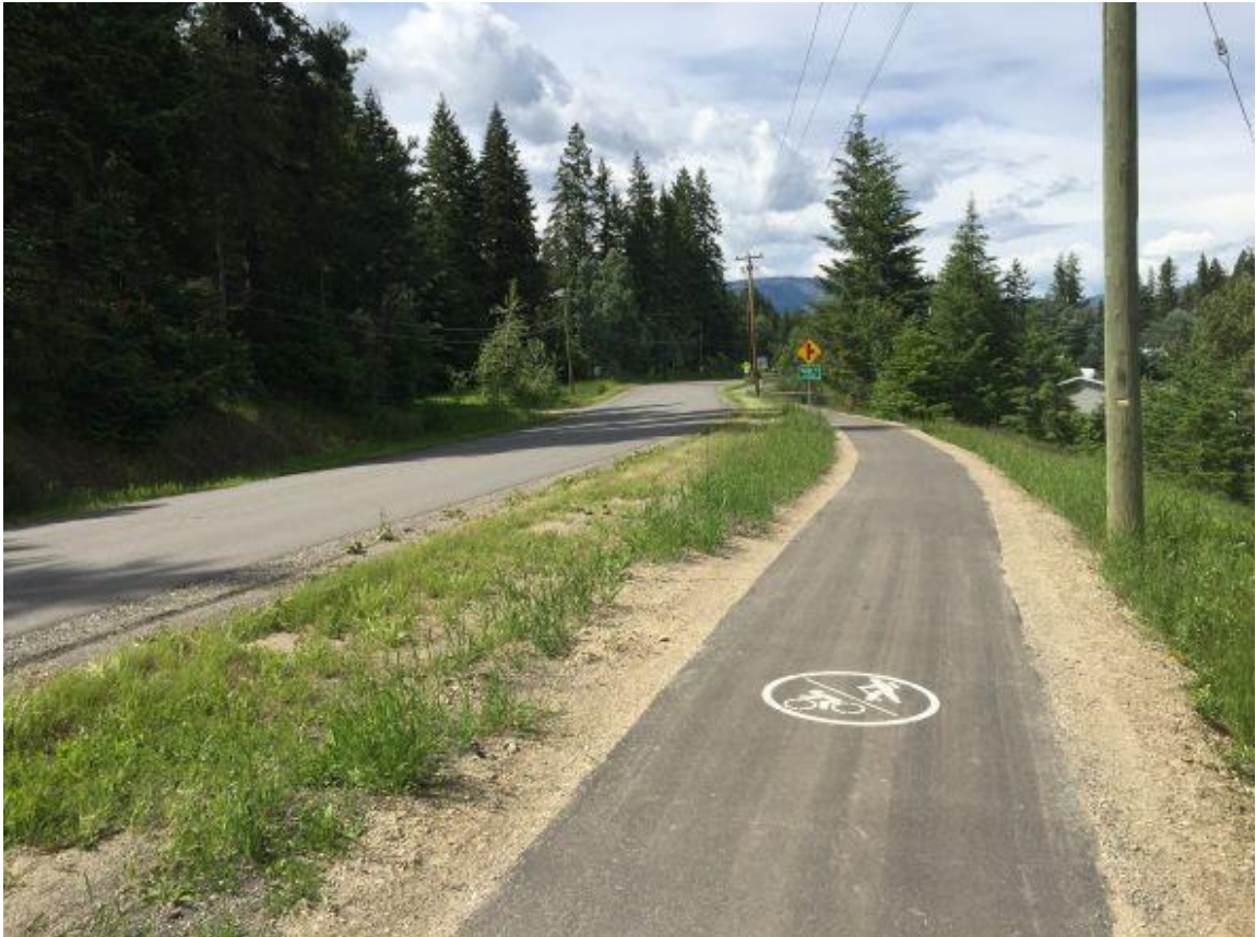
Example of asphalt surfaced option for community trail connections. (Salmon River Road)
