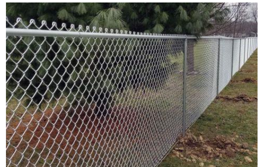
6' chain-link security fence.
