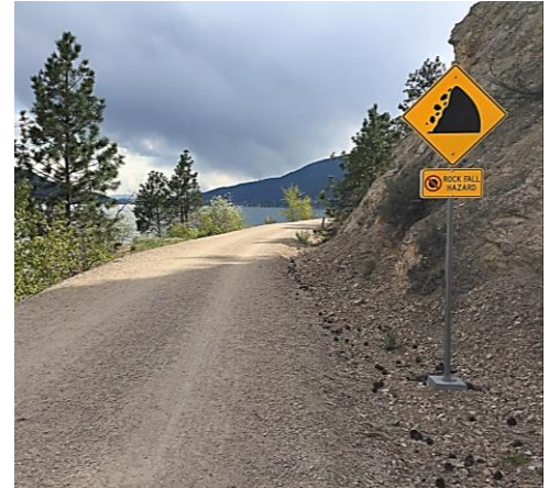
Rock Fall Hazard (Okanagan Rail Trail)
