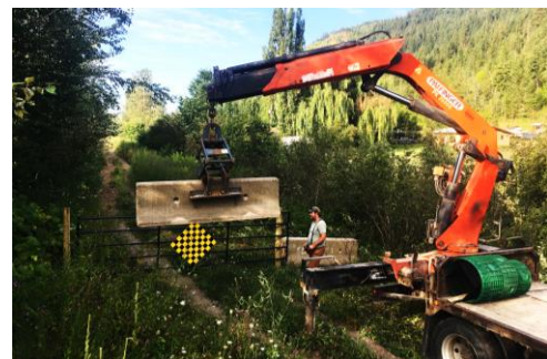
Concrete barriers. (Coell-Jones Rd, Mara)
