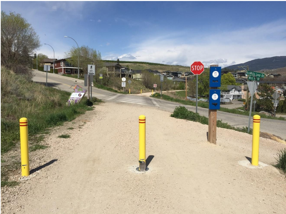
Bollards at trail entry points. (Okanagan Rail Trail) NOTE: SNO Rail Trail to include asphalt apron.
