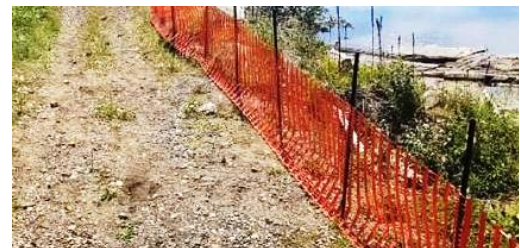
Temporary fence & T-Post. (SNO Rail Trail)
