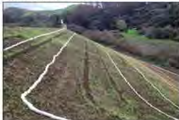
Filtrex SiltSoxx NATURAL ORIGINAL used as Slope Interruption.
